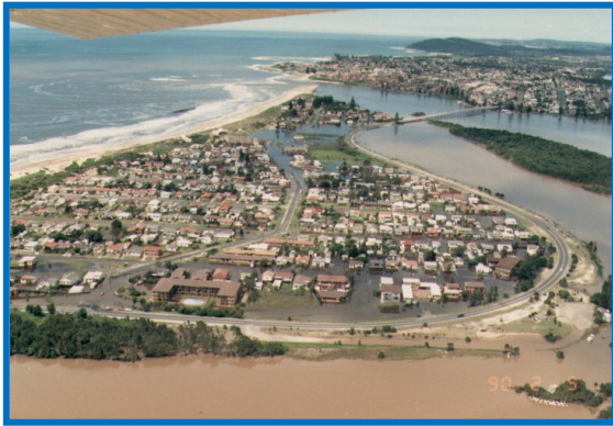
Entrance channel - February 1990 flood
