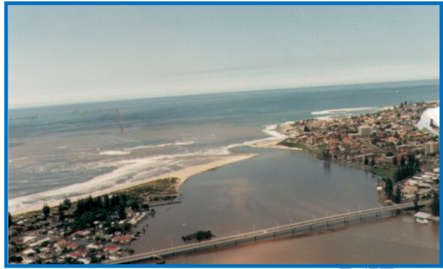
Entrance channel – June 2007 flood
